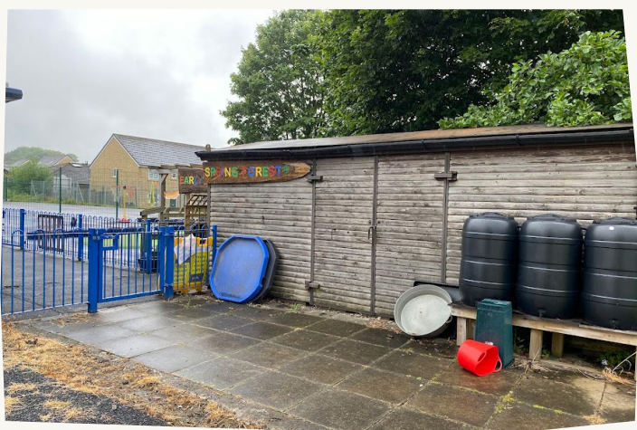
Shed before green roof
